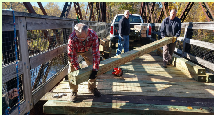
Moving timbers into place.
