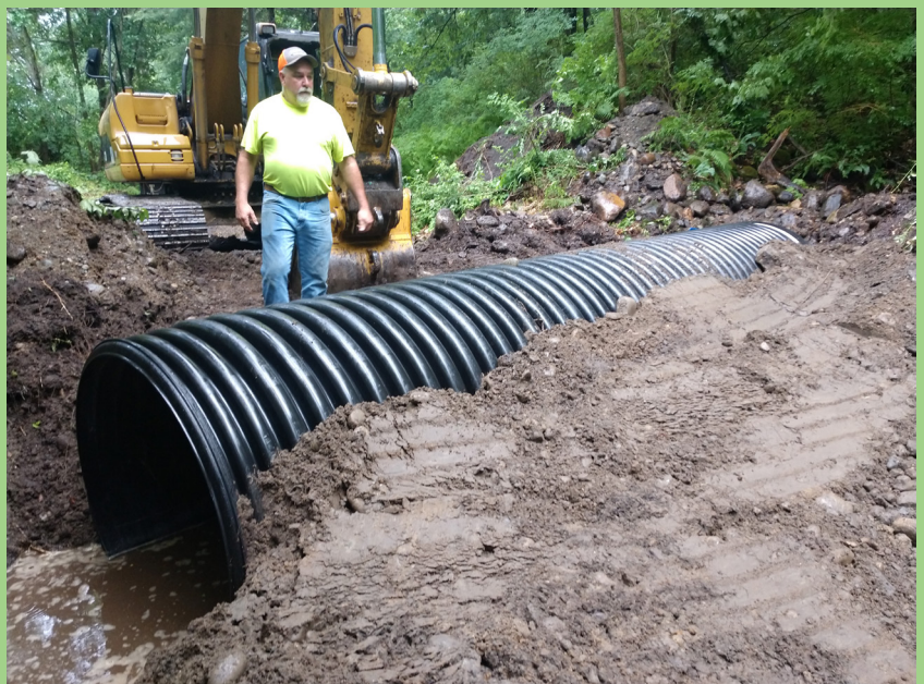
Weston inspecting the 48" culvert as he installs it.
