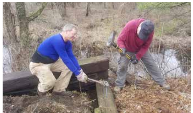
Mark and Mike pounding rebar into timbers for the picnic area.
