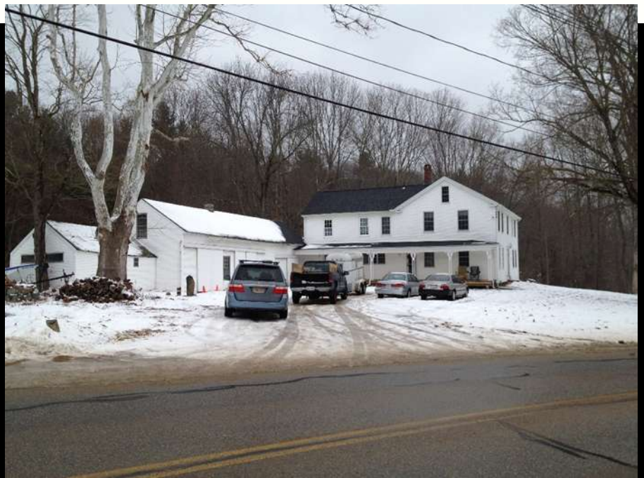
93. A typical arrangement of rooms in a farmhouse Erastus True Farm, North Yarmouth, Maine, built 1842.
