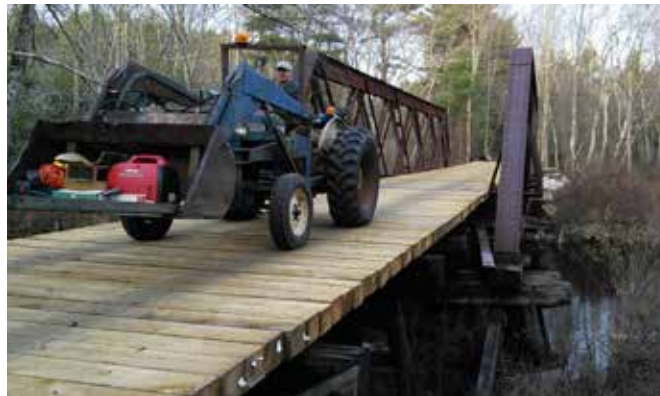
Mark with his tractor at the pony truss after finishing the decking repairs.
