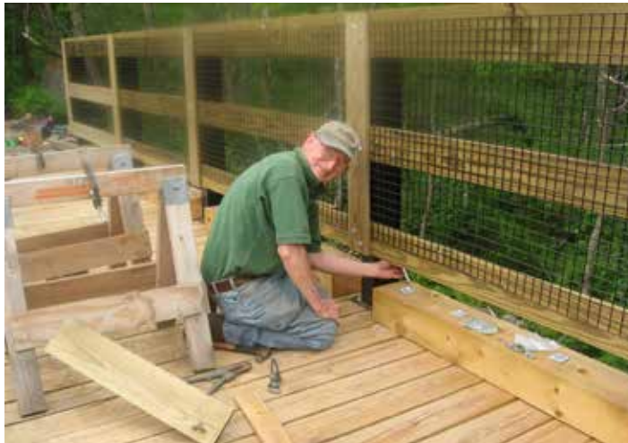
Ed Yaglou installing railing sections at the lattice truss bridge.
