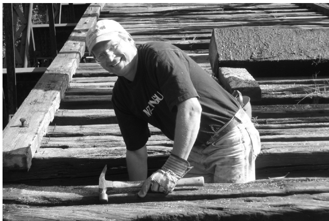
Mark Mattson emerging from the underside of the bridge after installing new blocks on top of the double bents.
